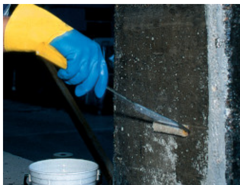
Applying MapeWrap 31 with a roller on the still fresh MapeWrap 11 (or MapeWrap 12)
